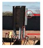
**Recognize the Hazard:** Meter and Riser installed, an Electrical Hazard exists!
