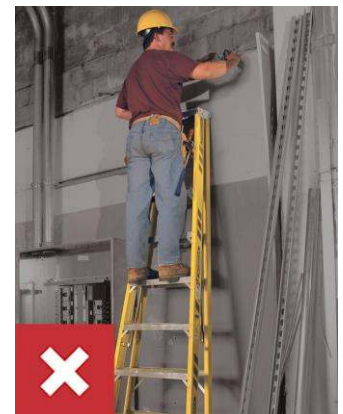
WRONG DON'T climb a closed ladder, it may slip out from under you.
