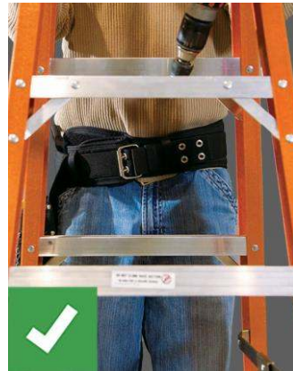
RIGHT Center body on the ladder and keep belt buckle between the rails while maintaining a firm grip.
