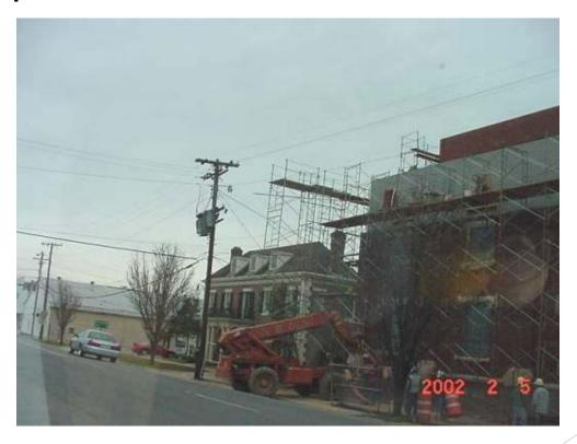
Keep 10 foot minimum unless de-energized, Relocated, or installed protective covering installed!
