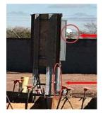
**Recognize the Hazard:** Meter and Riser installed, an Electrical Hazard exists!
