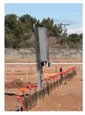
It is extremely important is to inform and educate onsite workforces about the hazards of energized Electrical Panels. The panel will be placed in its permeant position long before the house is built. The panel will be supported by 2 metal legs. These legs will remain in place and be out of sight once the house is nearing completion.
