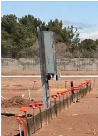
*It is extremely important is to inform and educate onsite workforces about the hazards of energized Electrical Panels. The panel will be placed in its permeant position long before the house is built. The panel will be supported by 2 metal legs. These legs will remain in place and be out of sight once the house is nearing completion.*
