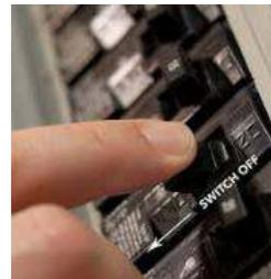
*All Panel Breakers and Main Breaker will be placed in the off position. (By the electrical provider APS/SRP). Builder to turn on breaker and verify temporary power outlets functioning prior to Lock-out / Tag-out.*
